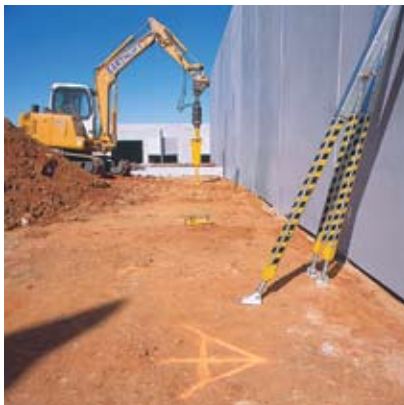
1. Plan and mark the location of each brace anchor on site.
